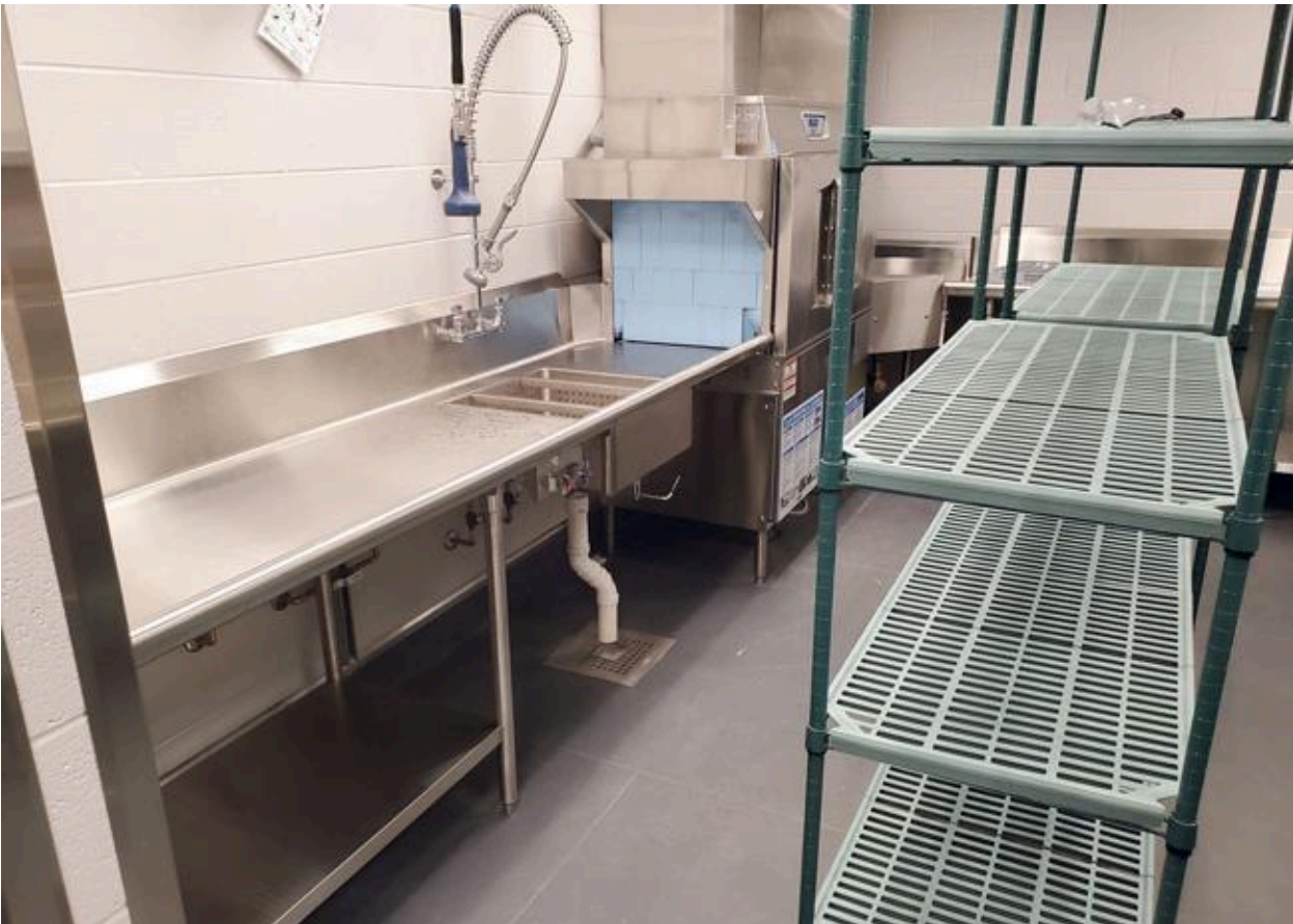
A corner conveyor and mobile shelving create a U-shaped dish room to maximize table space and utensil storage.
